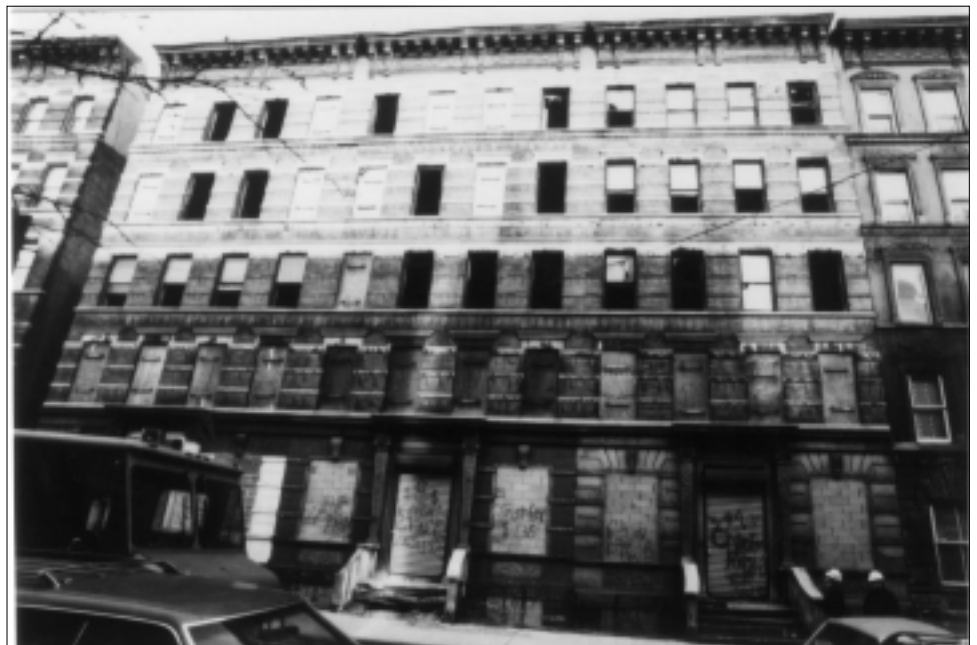
Before and after photos of Abyssinian House, a 25-unit rehabilitated apartment complex for formerly homeless families in New York City. Abyssinian Development Corporation of Harlem is one of New York's most prominent faith-based community development groups.
