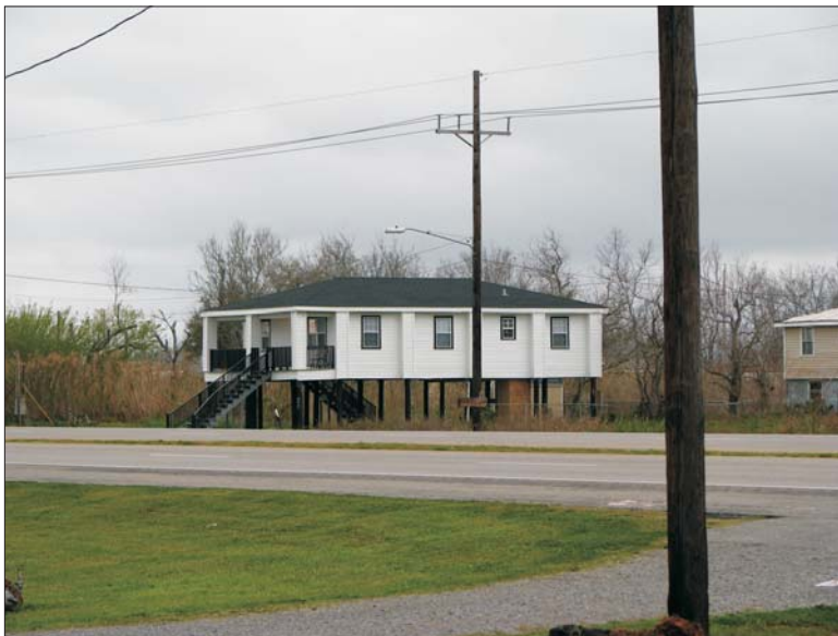
Elevated home built after Hurricane Katrina south of New Orleans, Louisiana.
