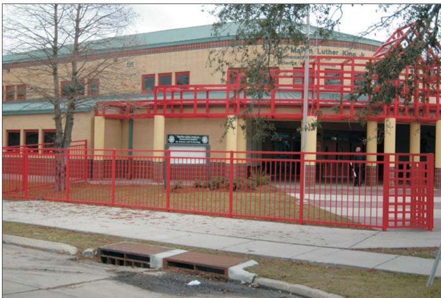
The repaired Dr. Martin Luther King Jr. Charter School for Science & Technology in New Orleans, Louisiana.
